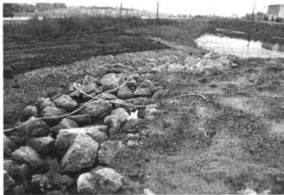
Channel from east inlet to pond
