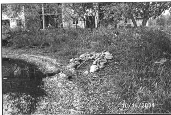
Inlet pipe looking northwest
