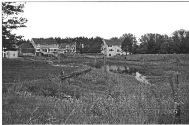
Pond looking south - erosion in foreground
