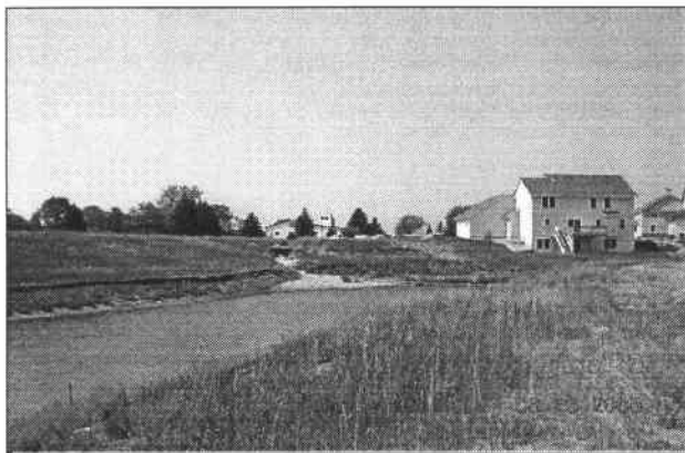
Erosion at southwest corner
