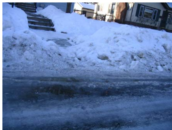
Zenith Ave with pooling water
