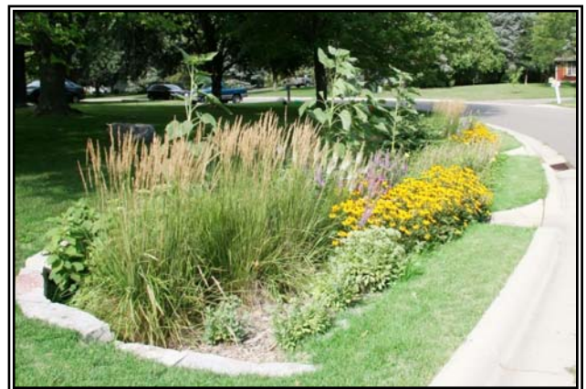
A curb cut rain garden.
