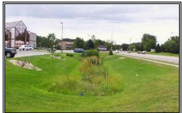
Typical infiltration swale
