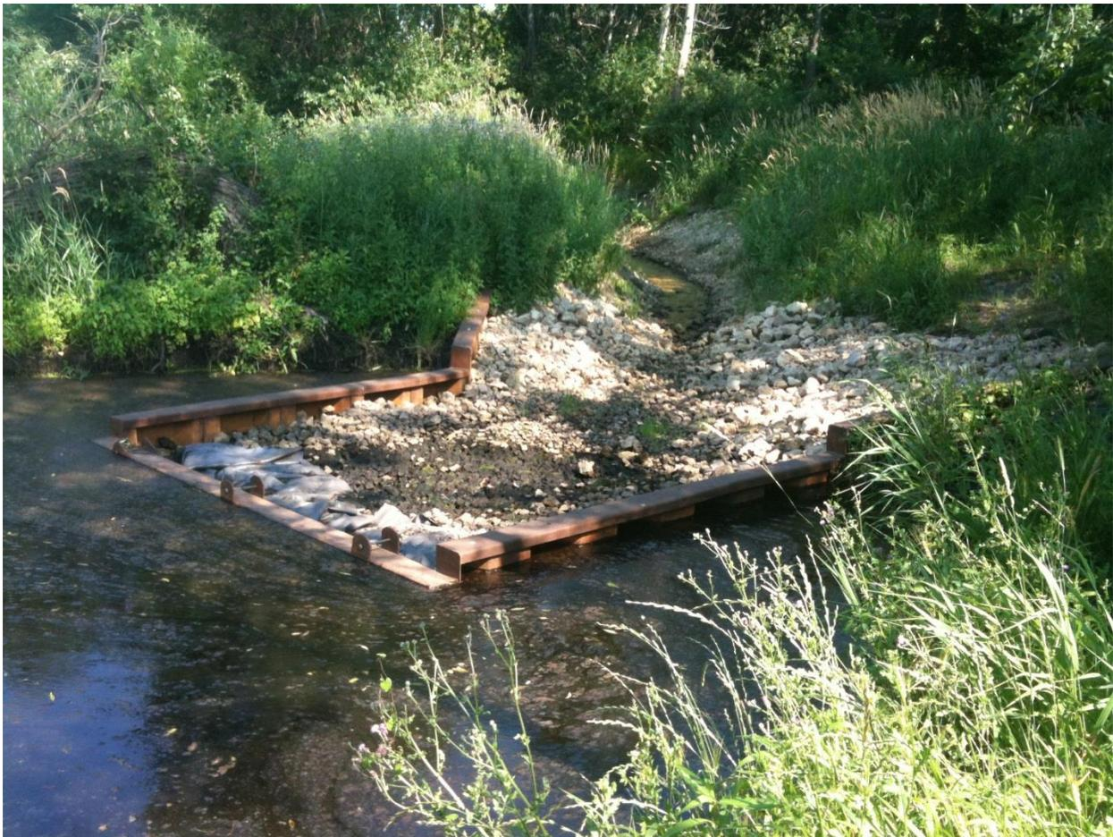
**Figure 1. The overflow weir at Wetland 639W.**
