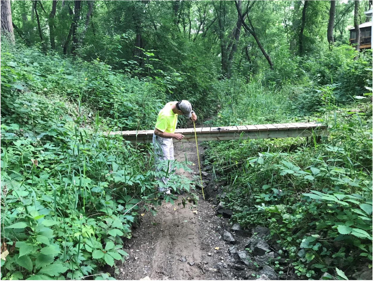
Small footbridge and typical conditions mid-reach.
