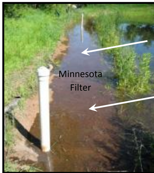
The two images show a Minnesota filter bench system before and after a storm event. As the pond fills with water from a storm it begins to enter the iron filter.
