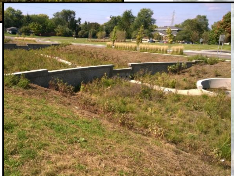
Pretreatment sump (at right) and concrete flume in Oakdale, MN
