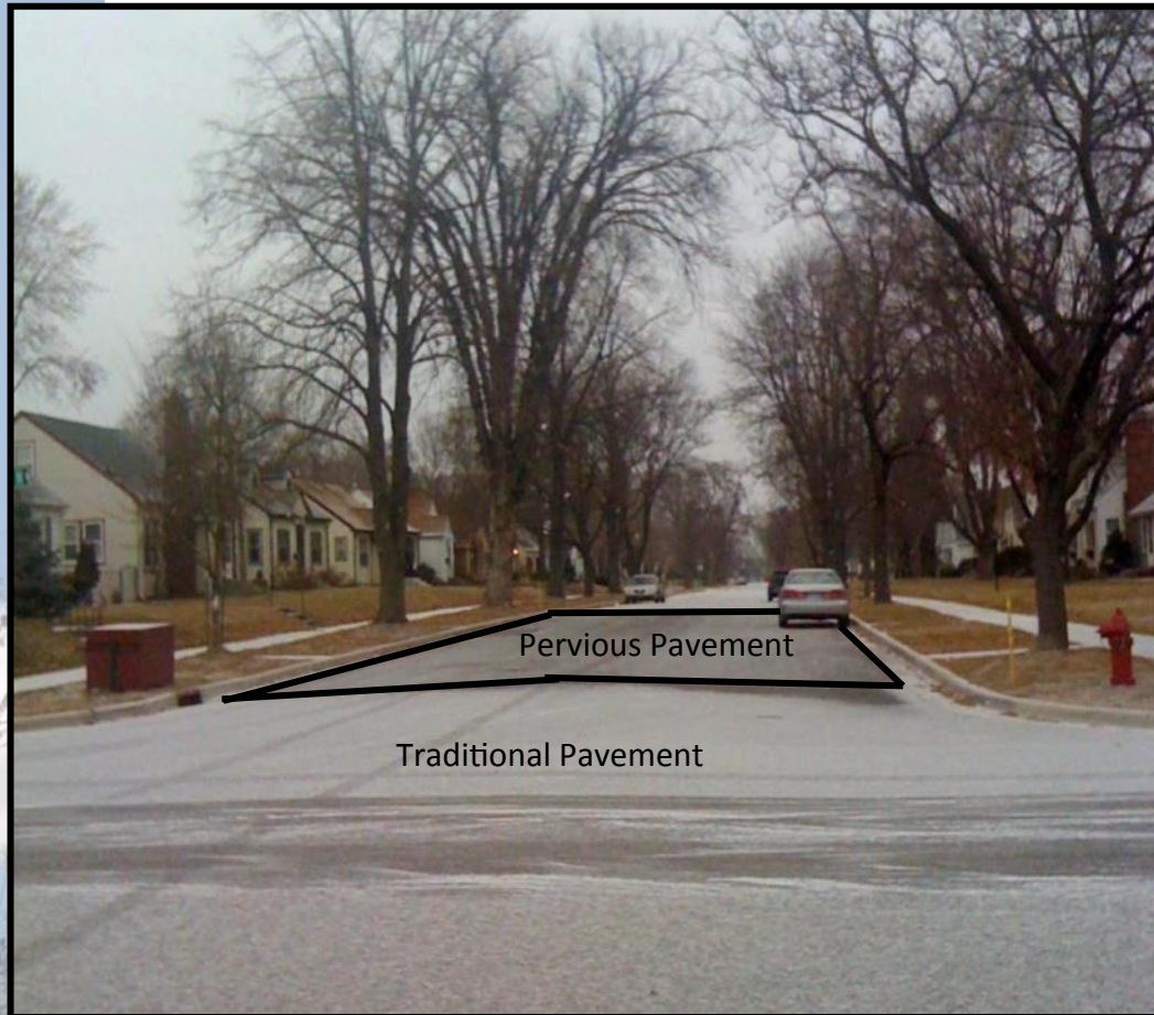
How snow accumulates on porous and traditional pavement in Robbinsdale, MN.
