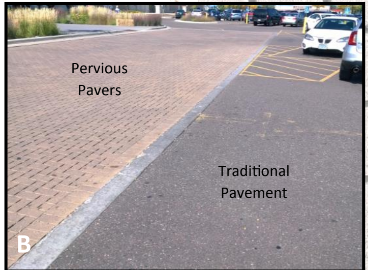
Images of pervious pavement in a parking lot (A) and low traffic areas (B).
