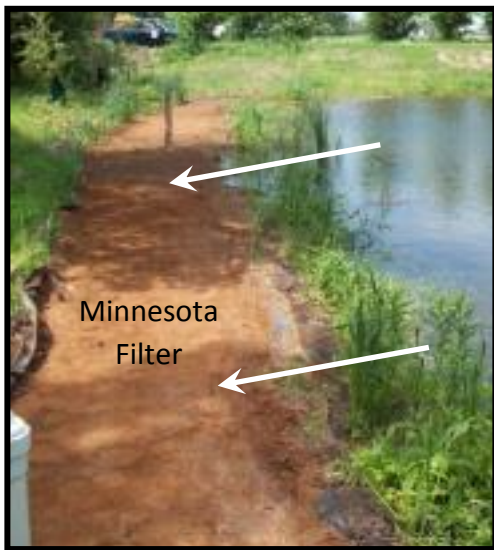
The two images show a Minnesota filter bench system before and after a storm event. As the pond fills with water from a storm it begins to enter the iron filter.
