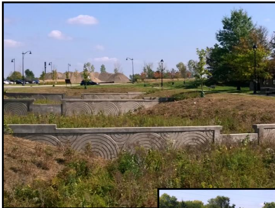
Bioretention “steps” in Oakdale, MN
