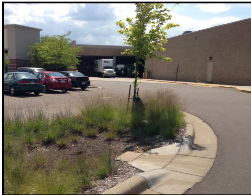
Island curb cut raingarden Maplewood Mall, MN
