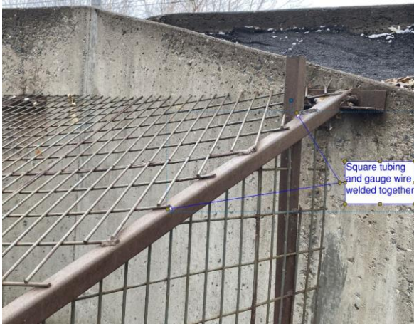
1 – Top part of cage is welded together.
