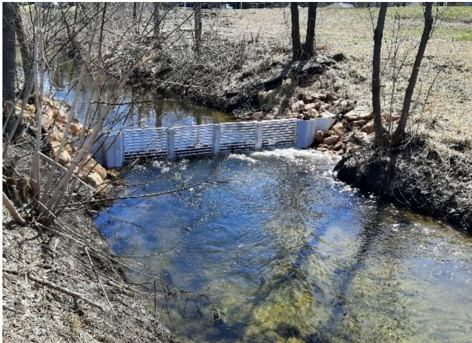
Figure 6. Horizontal bar fish barrier (image courtesy Rice Creek Watershed District).
