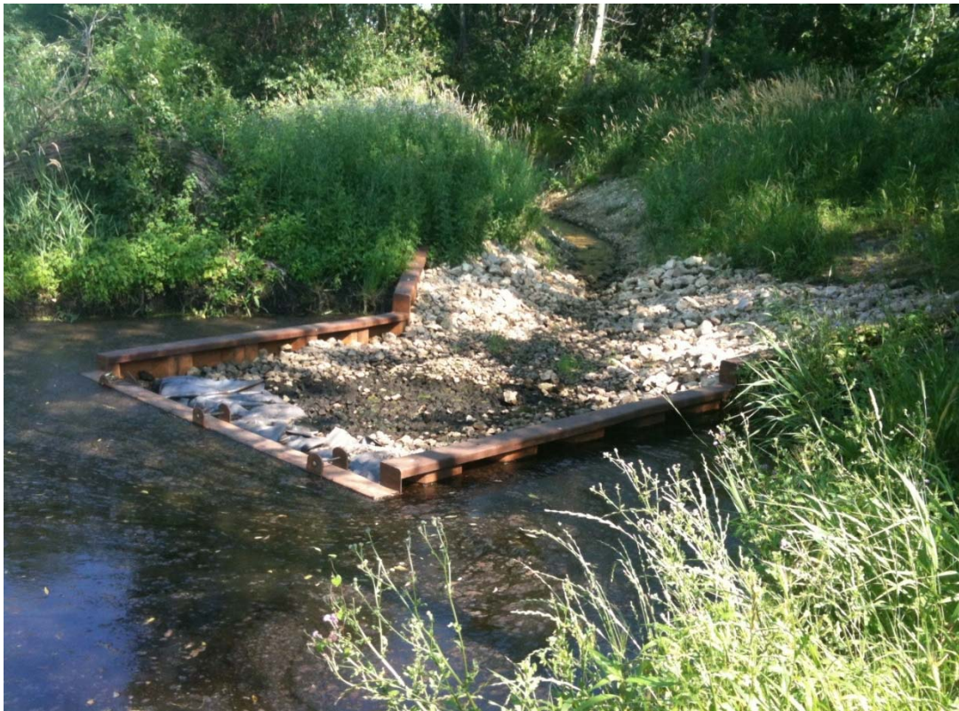
Figure 1. The overflow weir at Wetland 639W.
