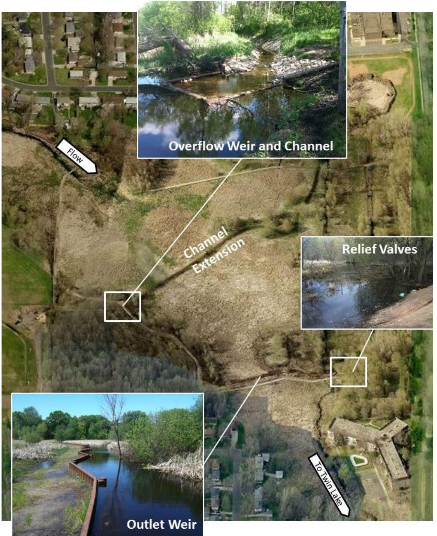
Figure 1. Wetland 639W outlet modification components.
