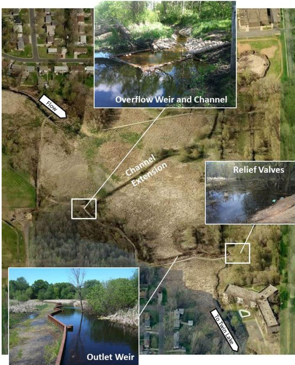
Figure 1. Wetland 639W outlet modification components.
